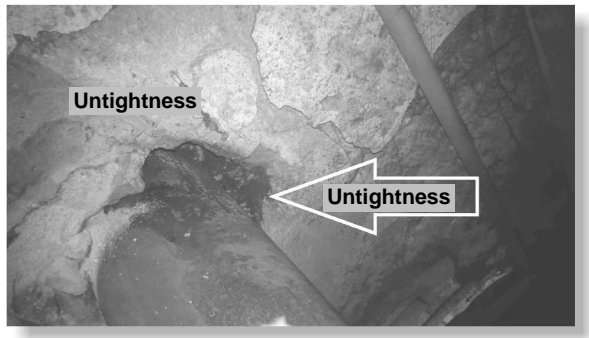
Wrong connection to the smoke uptake – it doesn't tighten and cannot be cleaned-up
