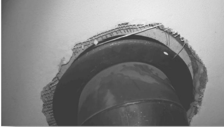
Wrong connection to the smoke uptake – it doesn't tighten and cannot be cleaned-up
