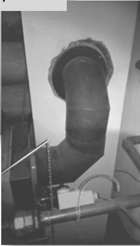
Wrong connection of the flue gas ducting and there is no dilatation of the smoke uptake
