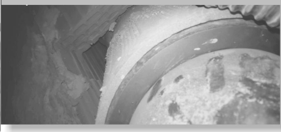
Wrong connection of the flue gas ducting and there is no dilatation of the smoke uptake
