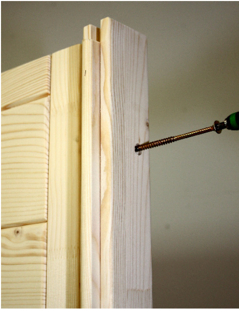
8 screws 6 x 120 mm per corner post
