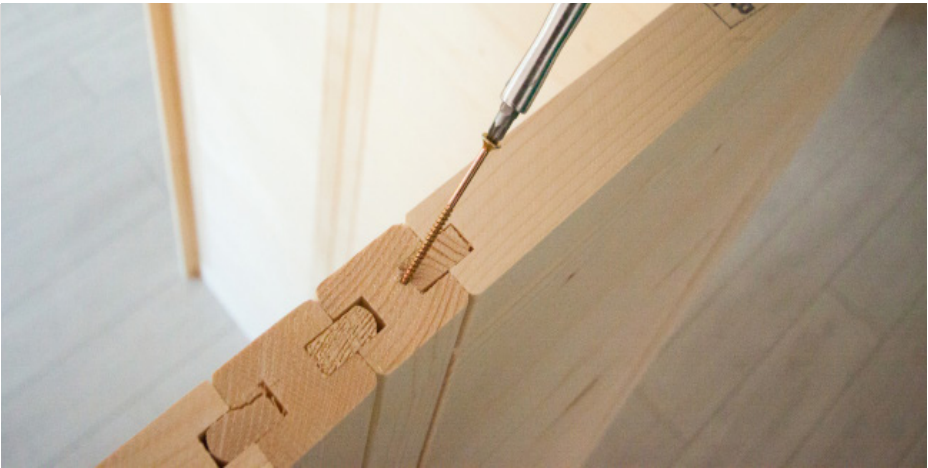
Foret de 3 mm, 17 vis 4 x 70 mm
