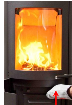
Fig. 5: adjust air lever
